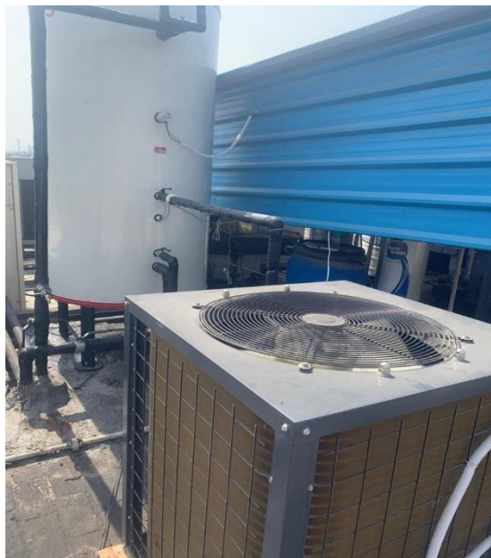
Figure 3-10: Use of heat pump
